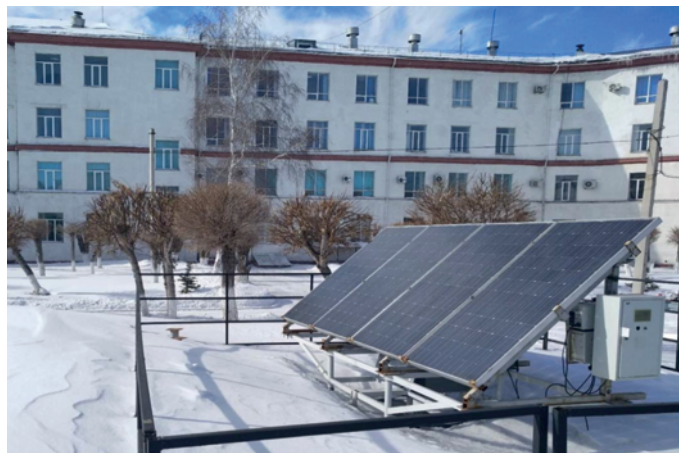
Fig. 2. The external view of SPP
